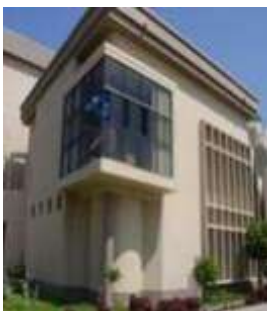
Vista exterior, zona central – UPAO
