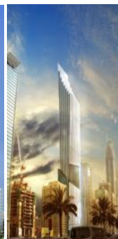
P-17 Tower, Dubai
